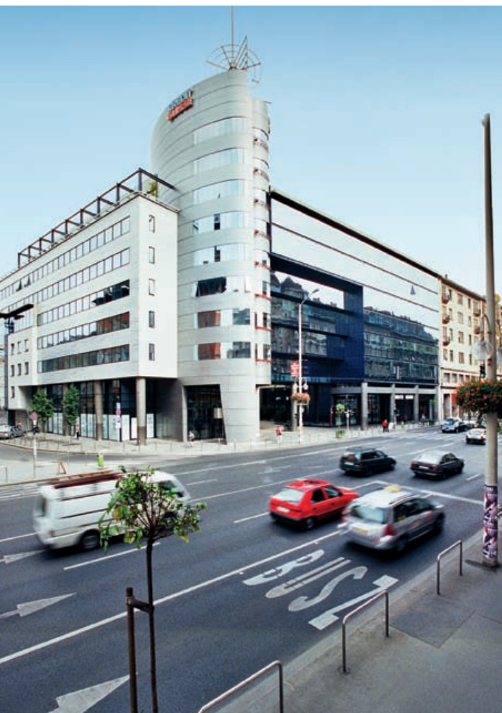
BUDAPEST R70 Office Complex
